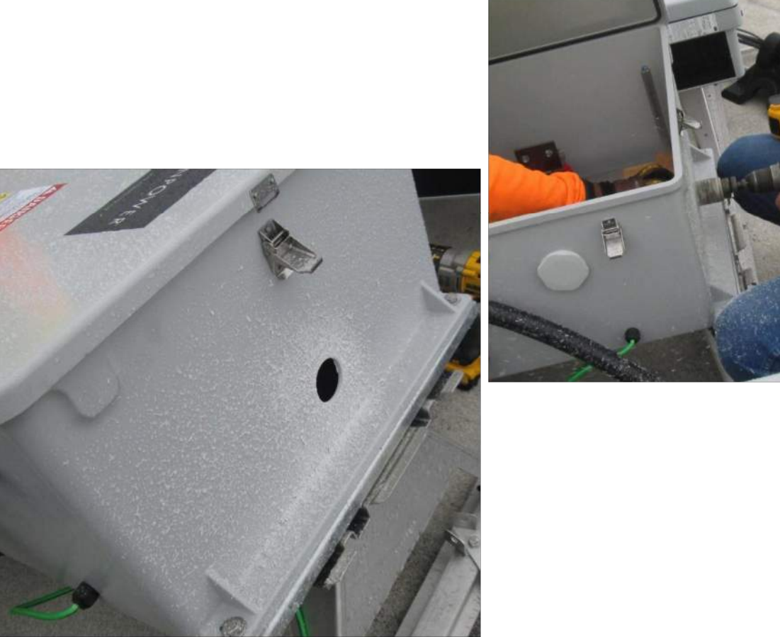
STEP A – DRILL CONDUIT EXIT INTO AC COMBINER
