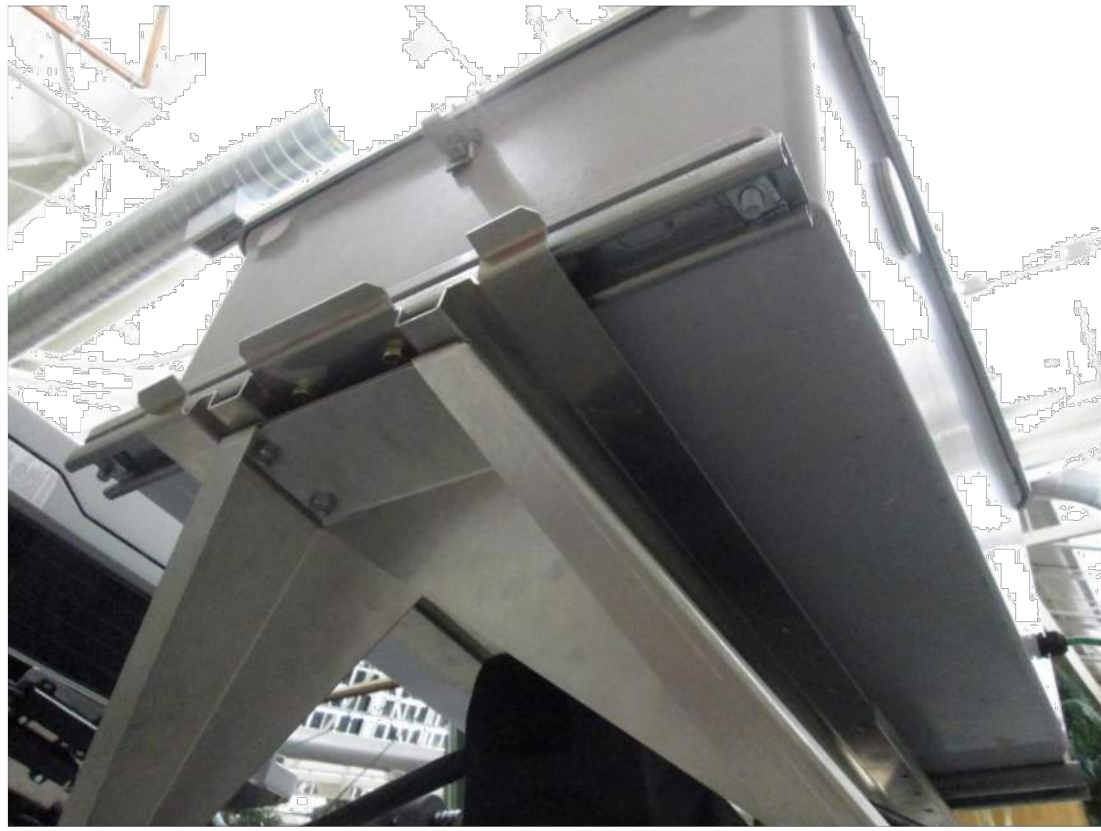
STEP D – SECURE AC COMBINER TO POWER STATION RACK
